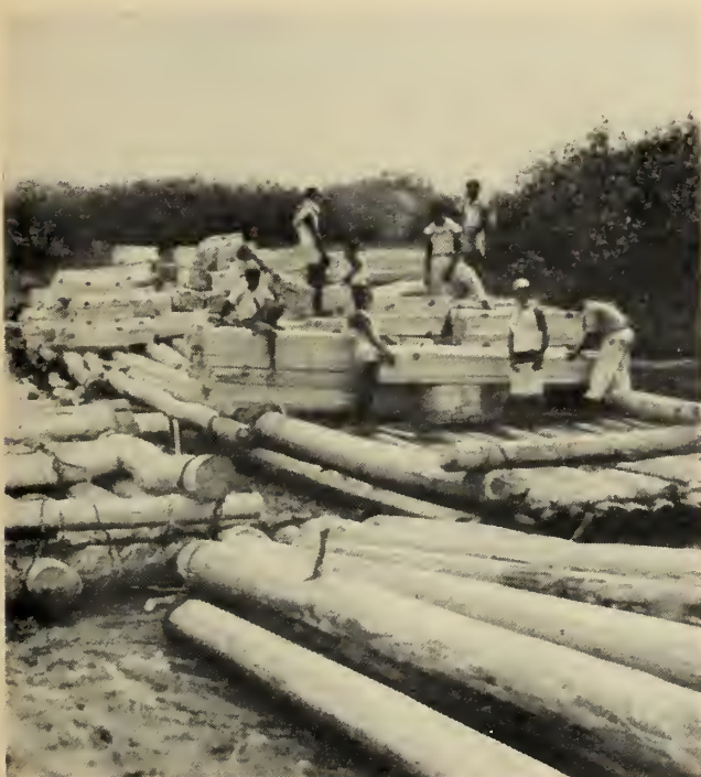
Loading lumber on balsa raft at the mill.
